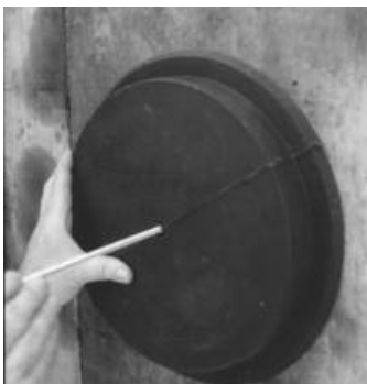
After nailing end cap to form, drive (threaded rod*) through the end plate and form and (thread nut*) on other side. Note: Remember to measure the (threaded rod*) to match the length of the sleeve.
